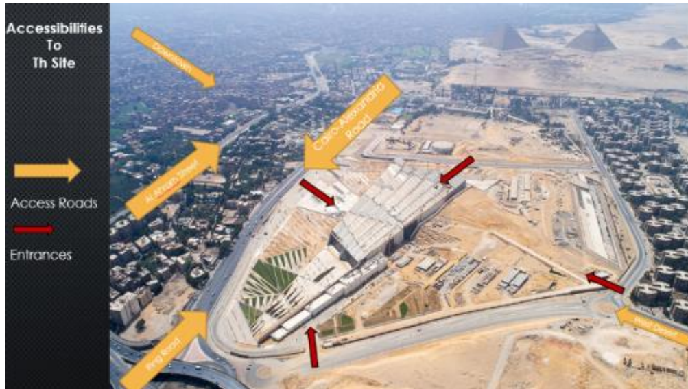
Fig 8: shows GEM museum accessibly, showing main entrance approach.
