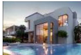
Figure15-2 Elevation-North Façade-source SODIC.com
