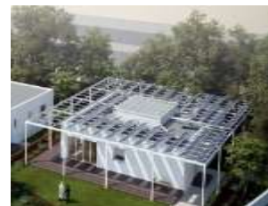
Figure 9 showing the PV cells array playing as a shading device, the light-colored coatings, and the west façade green walls.
