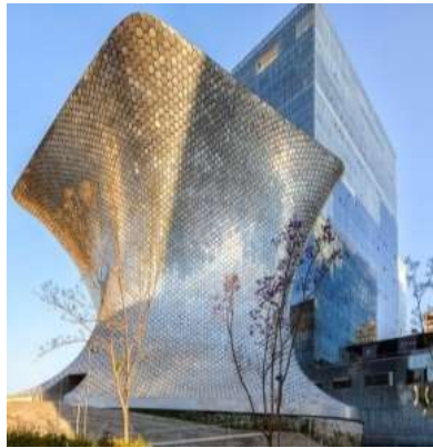
(b) Free form construction
