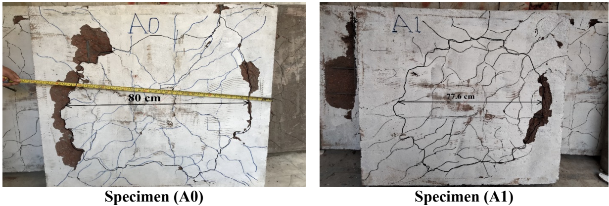
Fig. 12 The crack pattern in the tension side of all specimens.
