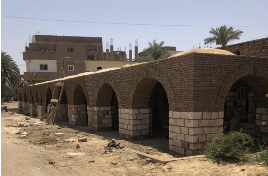
E: After remove the added exterior wall 2021.
