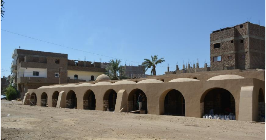
F: After the final restoration of the Khan 2021.
