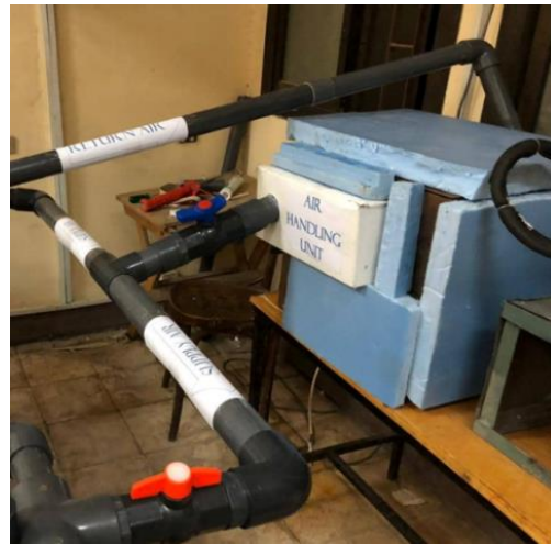
(b) AHU from outside
