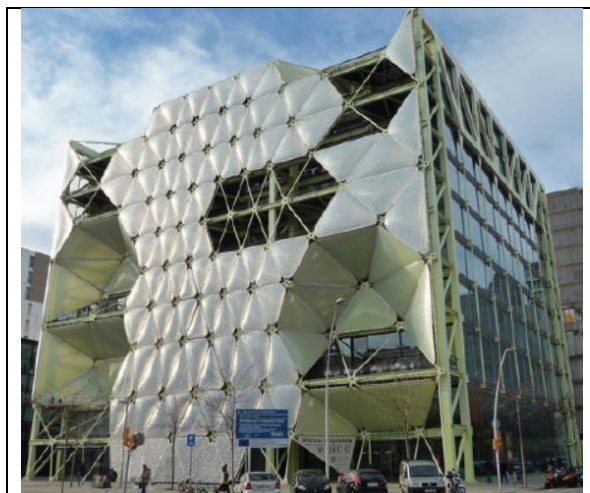
Figure 7 the media-tic office building 2011 in Barcelona, by cloud9, features a dynamic facade made of “breathing” ETFE air cushions (source:[4])
