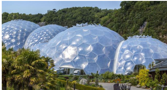
Figure 9 ETFE cushions used in the Eden Project
