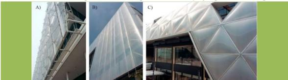
Figure 1 Double-skin façades with ETFE A) Unilever Headquarters in Hamburg, with single-layer clear ETFE; B) Tic-Media Building in Barcelona with double-layer ETFE cushion in south-west façade, C) Canary Wharf Crossrail Station in London with fritted double-layer ETFE cushion Source :(Pictures by J.-F. Flor, 2016/2017).
