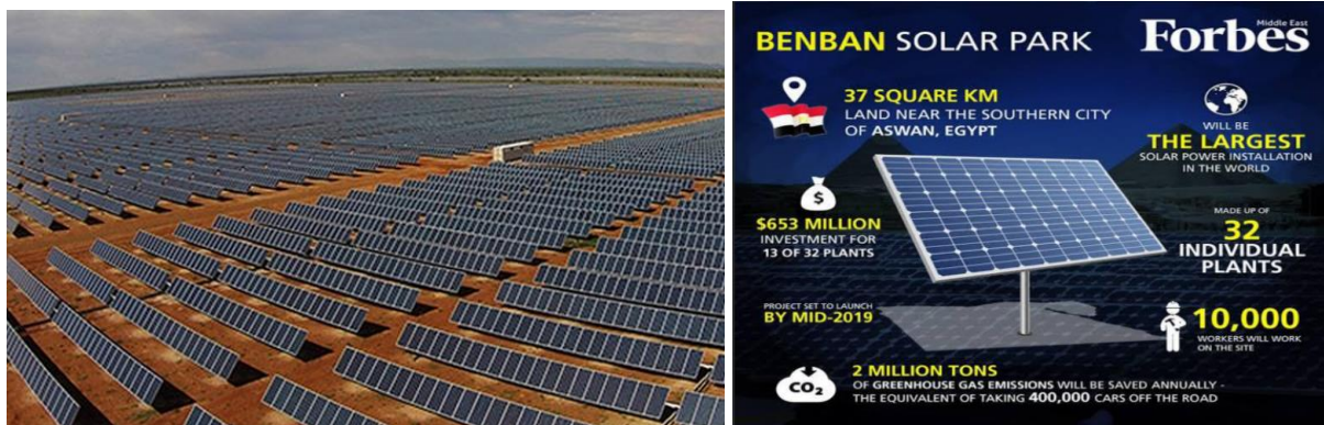
Figure(13) Benban", the Largest Solar Power Plant in Aswan
