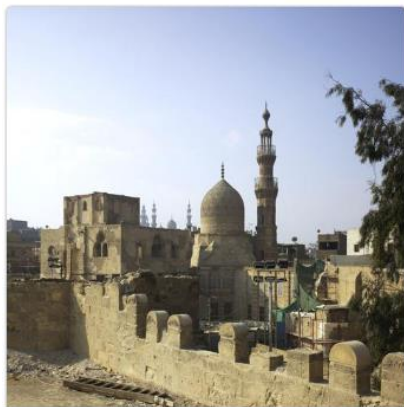
Ayyubid Historic Wall Conservation Cairo, Egypt
