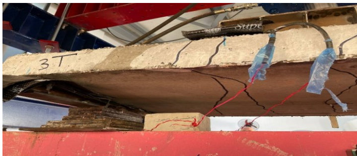
Figure 15. The Crack Pattern of Specimen ST350.
