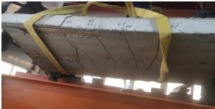
Figure 14. The crack pattern of Specimen SI350.
