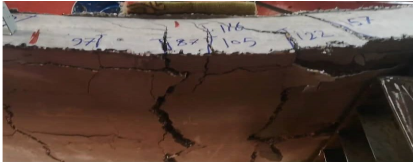
Figure 16. The Crack Pattern of Specimen SU350.
