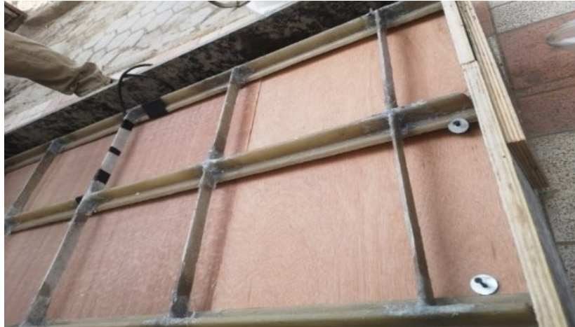
Fig. 10. Installation of the strain gauge in ST350S.
