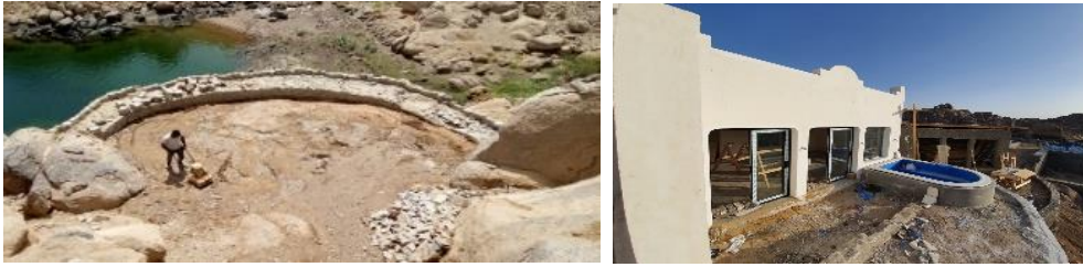
Fig. 5. The Rocky Ground at The Project Site Source: Mr. Tharwat Mohamed, the owner
