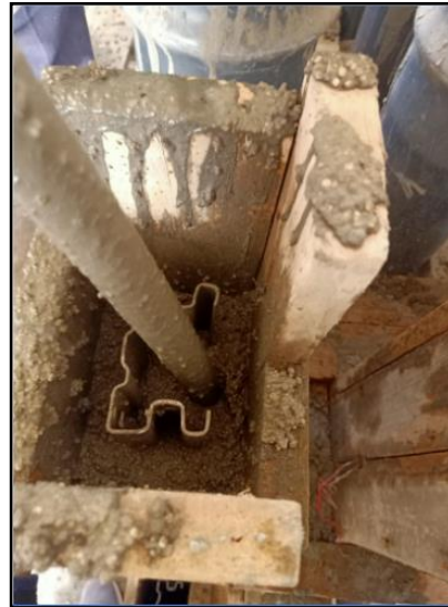
(b) Compaction of encased column
