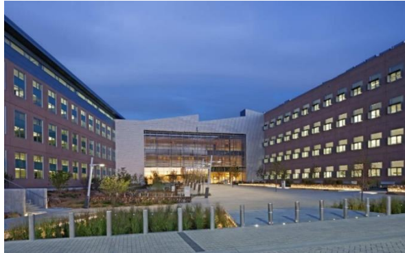
Figure23 shows Research Support Facility - United States Source: http://www.iaiotpen.org/node/ Accessed 20/4/2024
