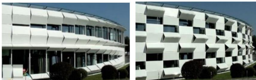
A figure13 showing the change in the facade shape of units in response to climatic conditions.
