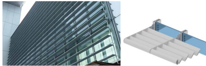
A figure6 showing the horizontal sun visors on the building.
