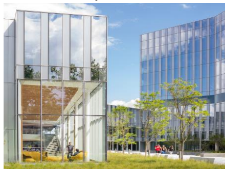
Figure 19 shows Radiation-permeable glass design with integrated sun breakers
