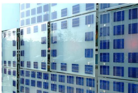
Figure16 shows the solar façades in the green building and the use of solar cells.
