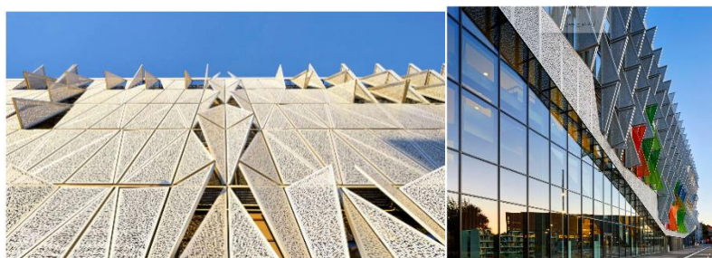
A figure15 showing dynamic facades. In SDU University of Southern Denmark Campus Kolding Source: https://arcdog.com/portfolio/sdu-university-of-southern-denmark-campus-kolding , Accessed 20-5-2024
