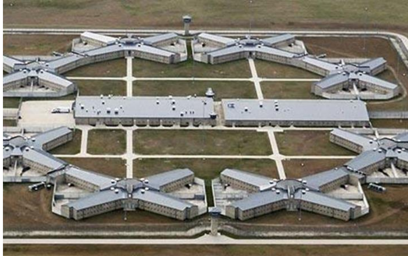
Fig. 12. The Administrative Maximum Security United States Penitentiary, ADX USP, Thomson, Illinois Source: https://morrisonchamber.com/about-morrison/bop-ausp-thomson/
