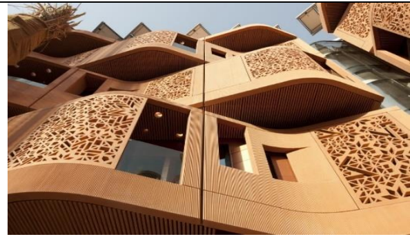
Fig. (9): The use of modern mashrabiya in residential facades Source: Reimagining The Mashrabiya: Functionality and Symbolism in Contemporary Architecture, March, 2024
