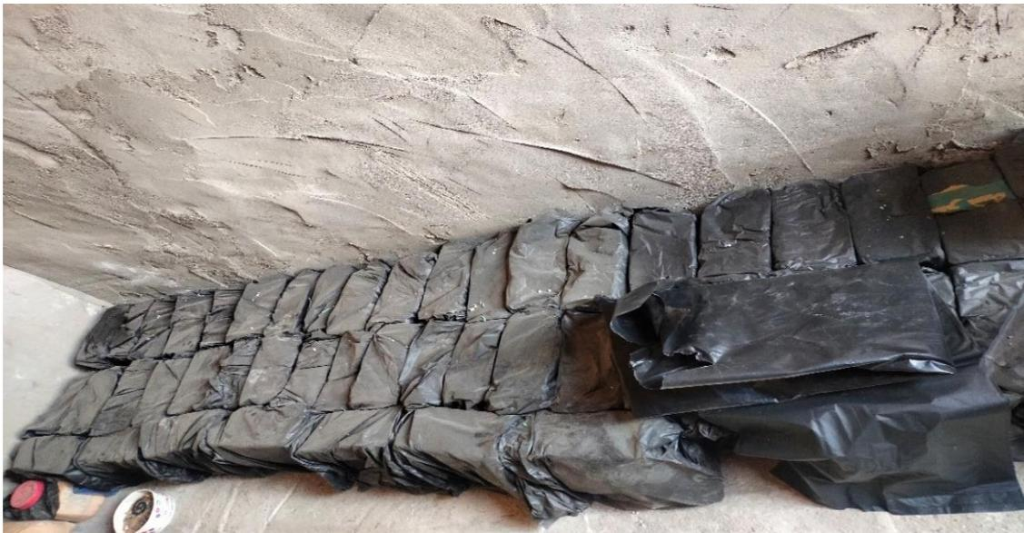
**Fig. 3:** Curing of Geopolymer concrete bricks in nylon bags 24 hours after casting for 7 days.
