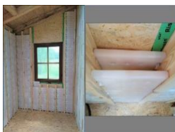
Fig. 16. Two-layer integration of PCM boxes in wall. [38]
